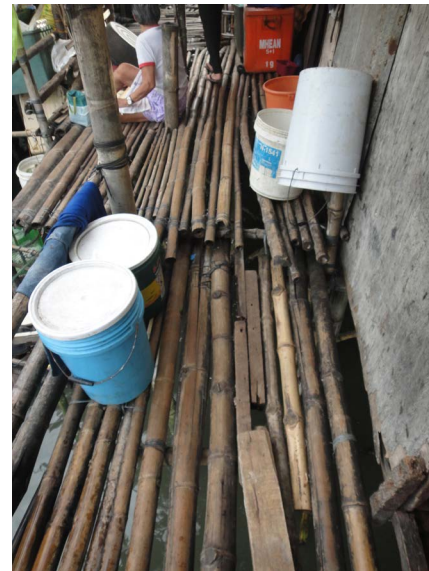
deck Huts are connected by boardwalks, shared decks and walkways made of bamboo. Used containers of petroleum, paint and other materials are reused for all utility purposes.
